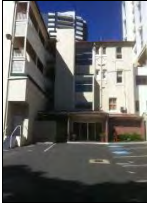
New rear entrance and elevator 2010.
